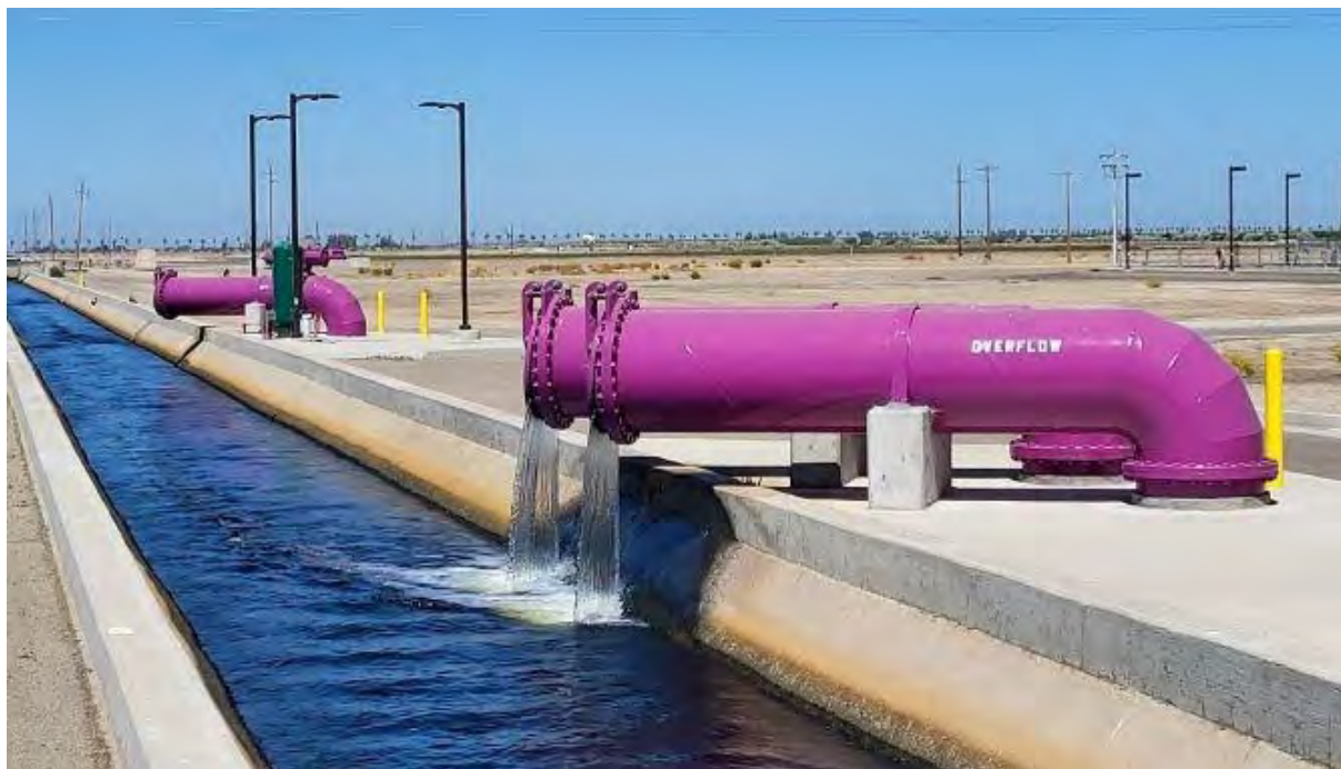
Photo 10. The City of Fresno Supplementing Water Supply Using Recycled Water, Indicated by the Purple Pipes
