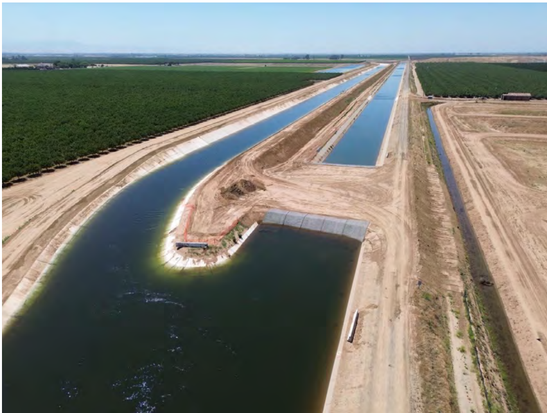
Photo 7. Friant-Kern Canal Middle Reach Capacity Correction Project Northern Tie-In with Existing Canal
