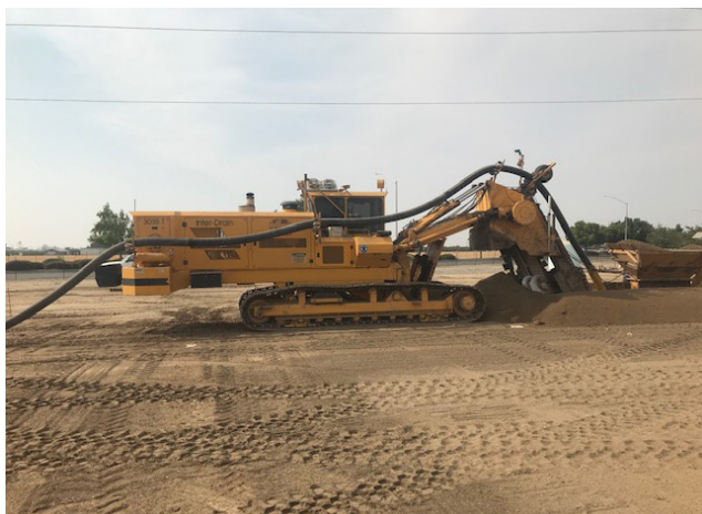
Figure 5 - Lidco excavator installing perforated SSAGR pipeline 1
