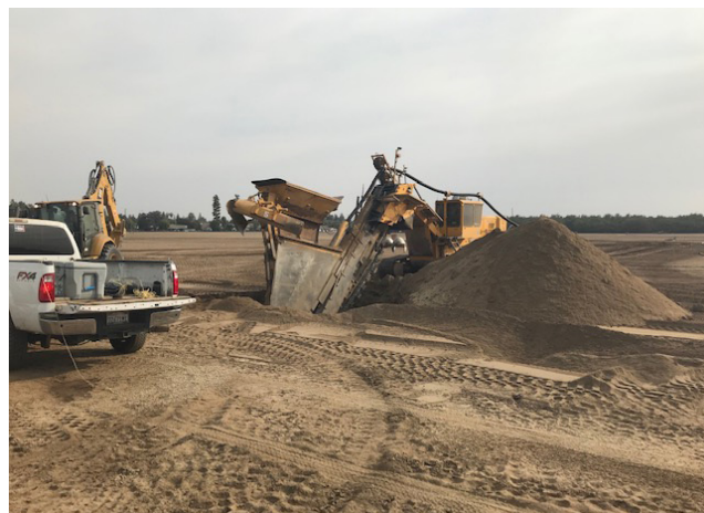
Figure 6 - Lidco excavator installing perforated SSAGR pipeline 2
