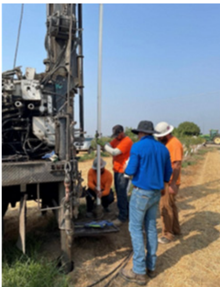
Figure 7 - Installation of a Moisture Probe Casing
