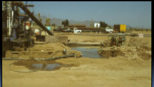
Reverse Rotary Rig and Mud Pit
